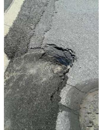
This sinkhole was a repeat, which ended up being the result of a corroded pipe as well.
