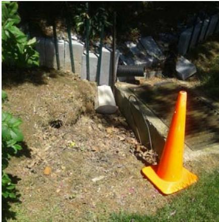
This sinkhole was caused by a pipe separating from the structure and allowing water in through a void.
