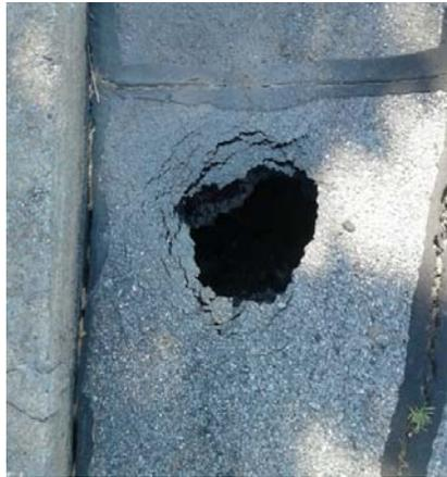
This sinkhole is the result of a corroded pipe which was exacerbated by hydrant flushing.
