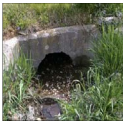
Figure 2: Sediment buildup
