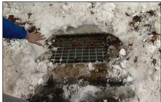
Figure 3: Clearing snow from Storm Inlets
