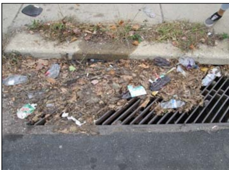
Figure 2: Trash & Leaf Litter on Inlet
