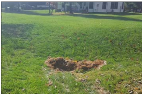
Figure 1: Pine Needles on a Yard Inlet
