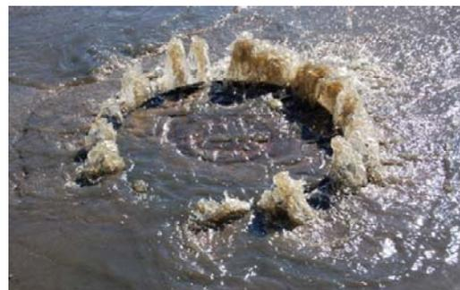
Figure 2: Liquid Sanitary Sewer Overflow
